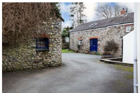
Entrance & Parking Area
