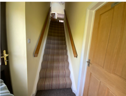
Entrance Hall & Stair To First Floor Landing
