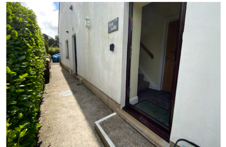
Path To Entrance Door
