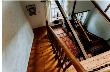
Stair to Second Floor
