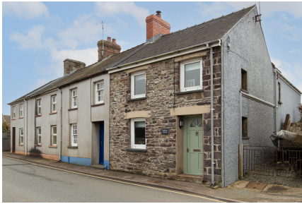
Street View & Entrance Door
