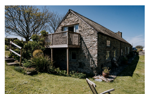
Bedroom 4 Balcony Terrace
