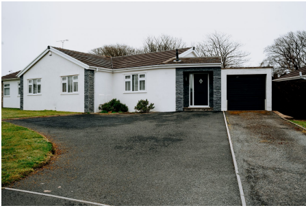
Driveway & Entrance Door
