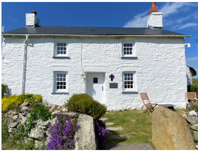
Front Door - Occasional Use
