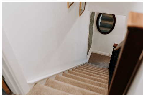
Stair to First Floor
