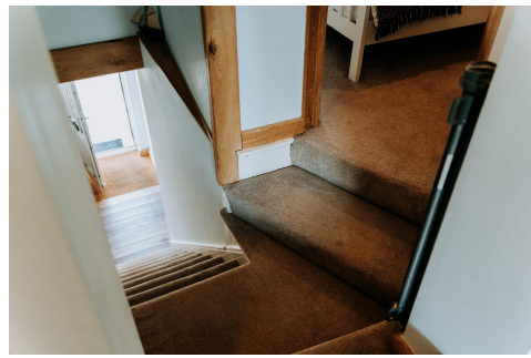
Stair to First Floor
