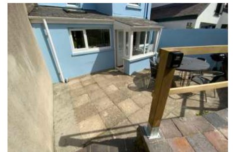
Rear Door To Porch & Key Box
