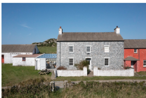
Farmhouse Wall Enclosure & Access
