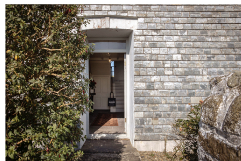
Entrance Door Threshold
