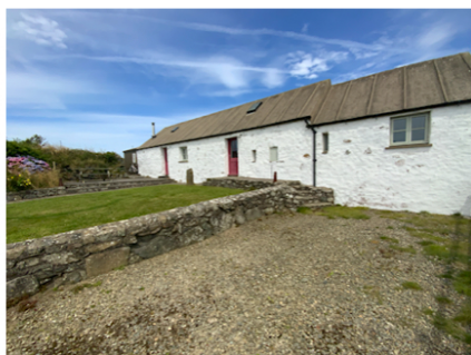
Gravelled Parking Area
