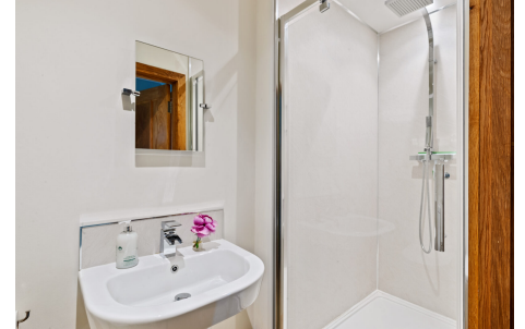
Ground Floor Shower Room
