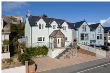
Parking Area & Ramped Access
